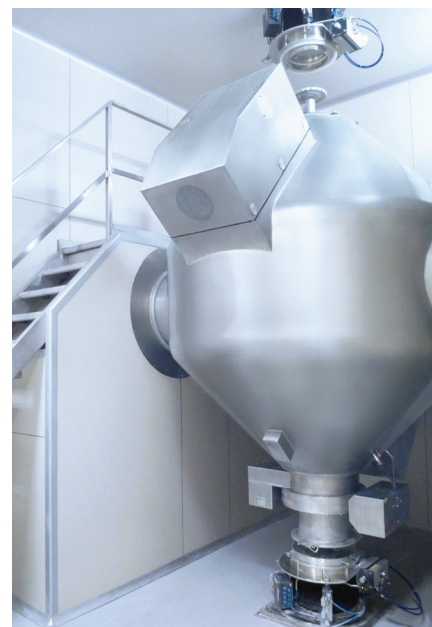
CRIOX Clean room installation (partitioning)
